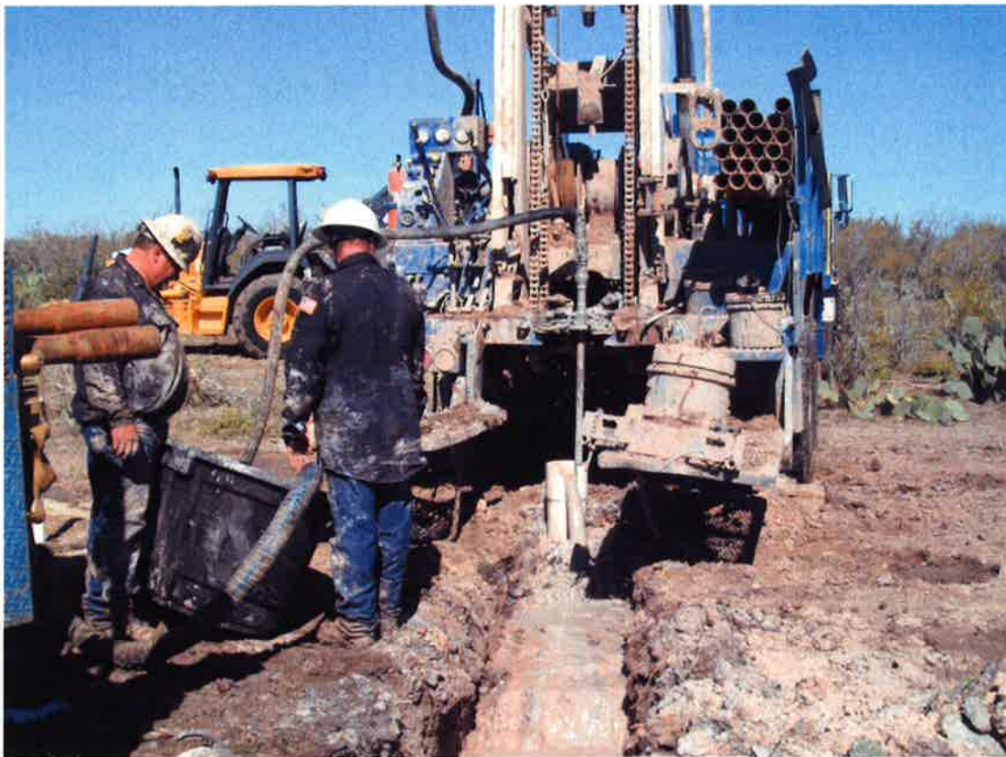
Photo 3 - Grouting Boring B-52 – January 2015
